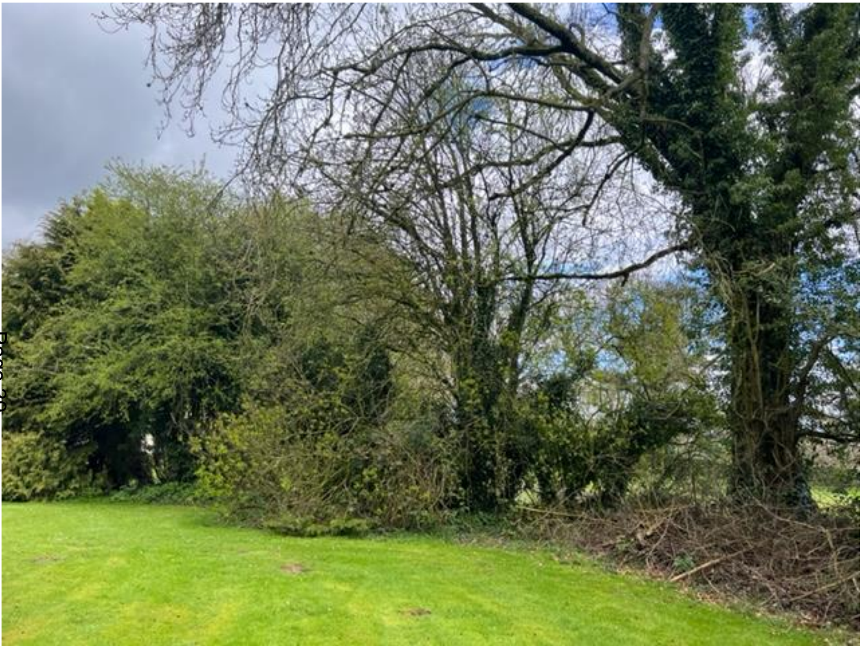
PART OF VEGETATION BOUNDARY BEING REMOVED FOR THE ACCESS ROUTE (FACING NORTH WITHIN THE SITE)
